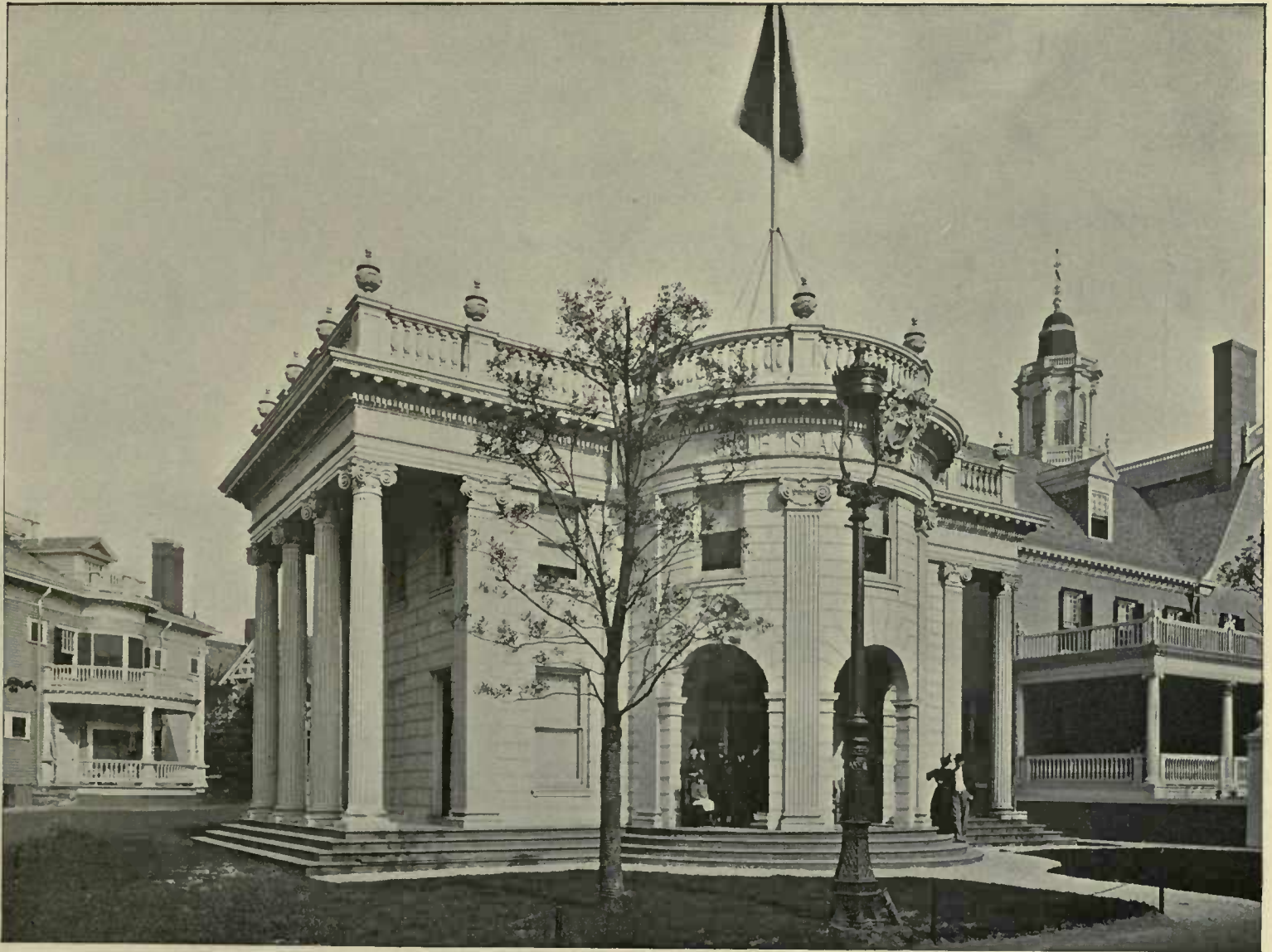
Rhode Island Building.
